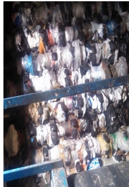
Plastic bags clogs separation equipment that employees have to clear
